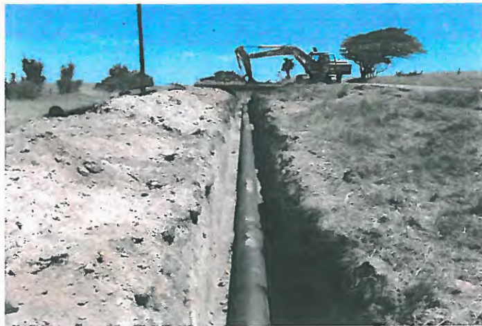
CONSTRUCTION OF A 350ØDUCTILE IRON PIPE AT USUTHU RWSS
